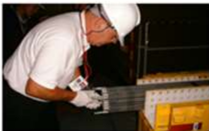
REPLACING UPPER TIE PLATE ON FUEL BUNDLE RODS AFTER REPLACING DAMAGED FUEL ROD IN BUNDLE
