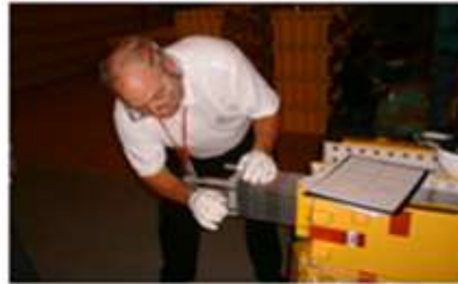
REPLACING HEX NUTS ON TIRE RODS
